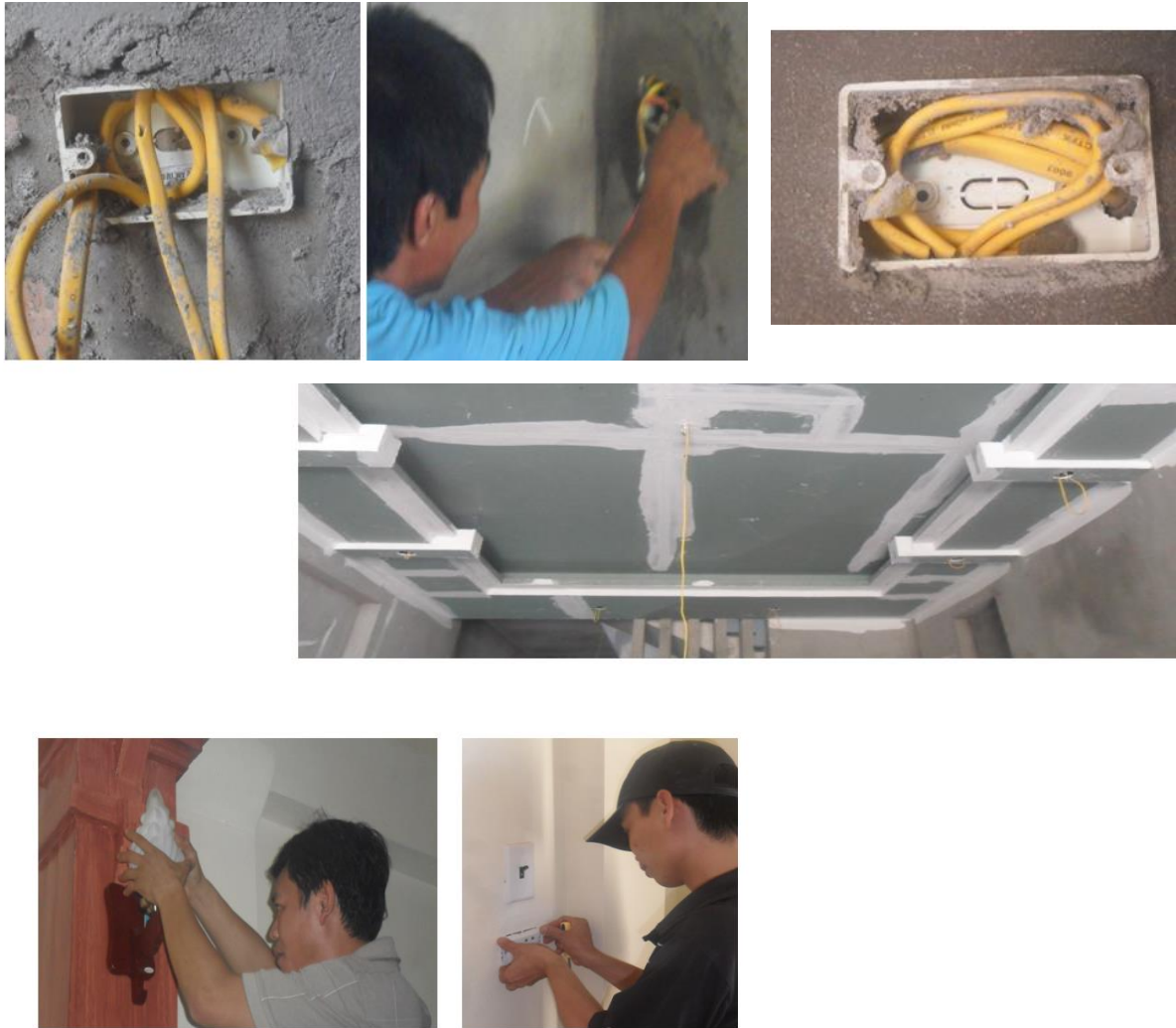
Electrical installation in process
